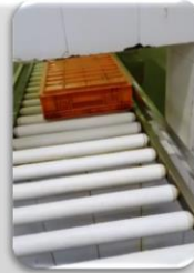
Tray & Conveyor Belt Sanitization
